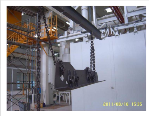
Shot blasting of Small structures
