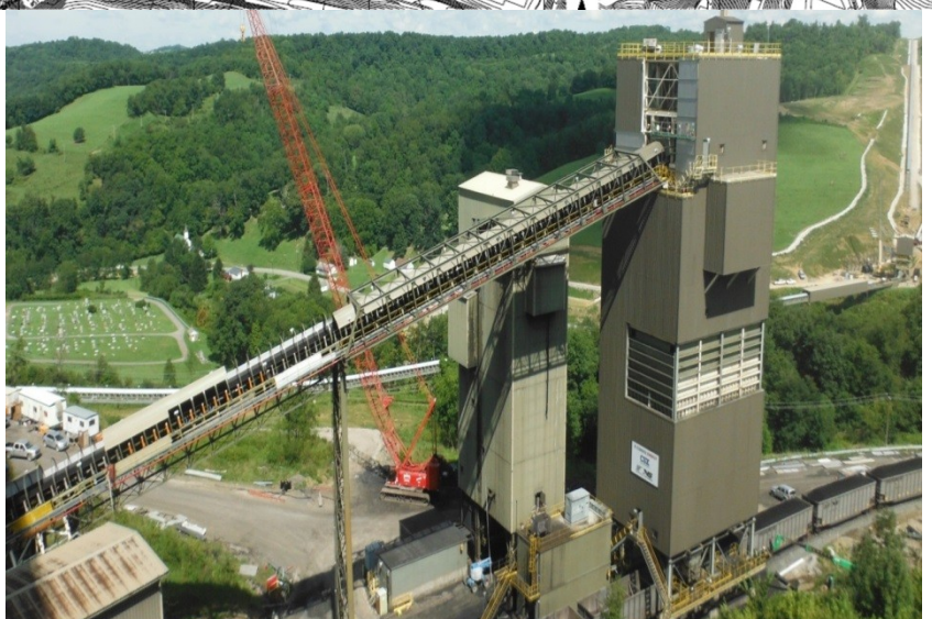
Upgrades to Prep Plant including New Dual Batch Train Load out Facility capable of loading 9,000 TPH and New 8,000' Rail Siding.
