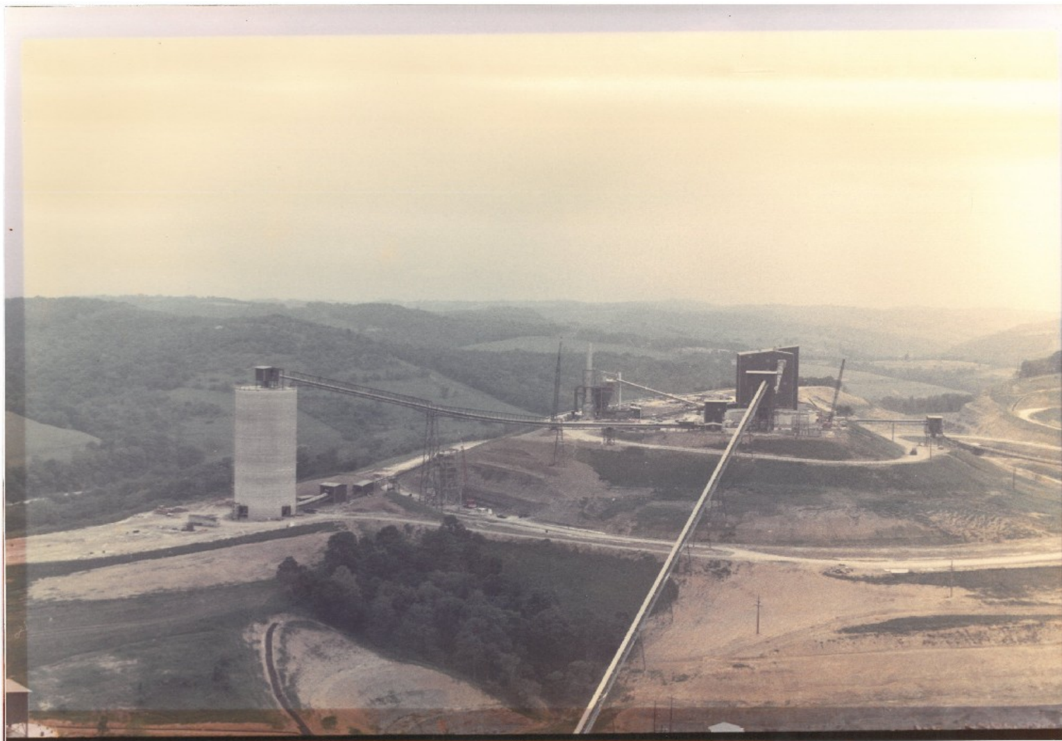
Bailey Preparation Plant 1984.
