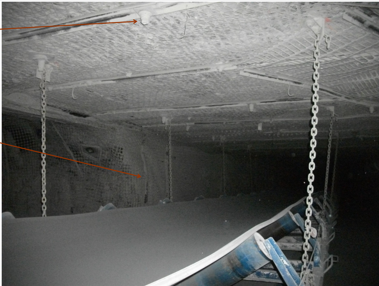
Harvey Mine life of mine main line haulage ground control.
