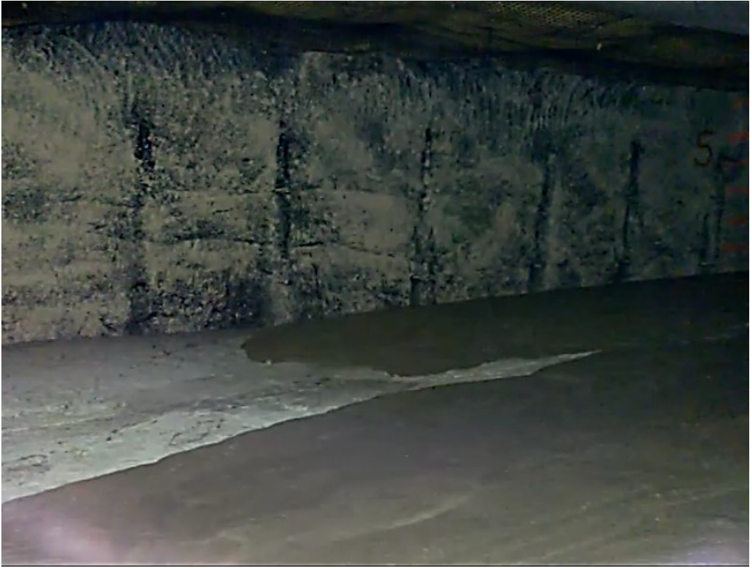
Backfilling 4 Right recovery room
