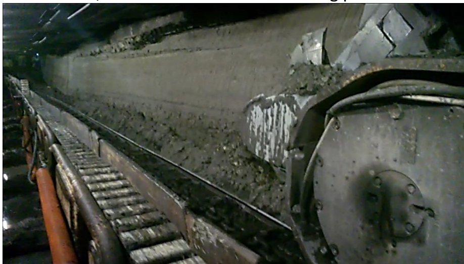
Mining the concrete backfill, no roof spalling. The face is standing straight.
