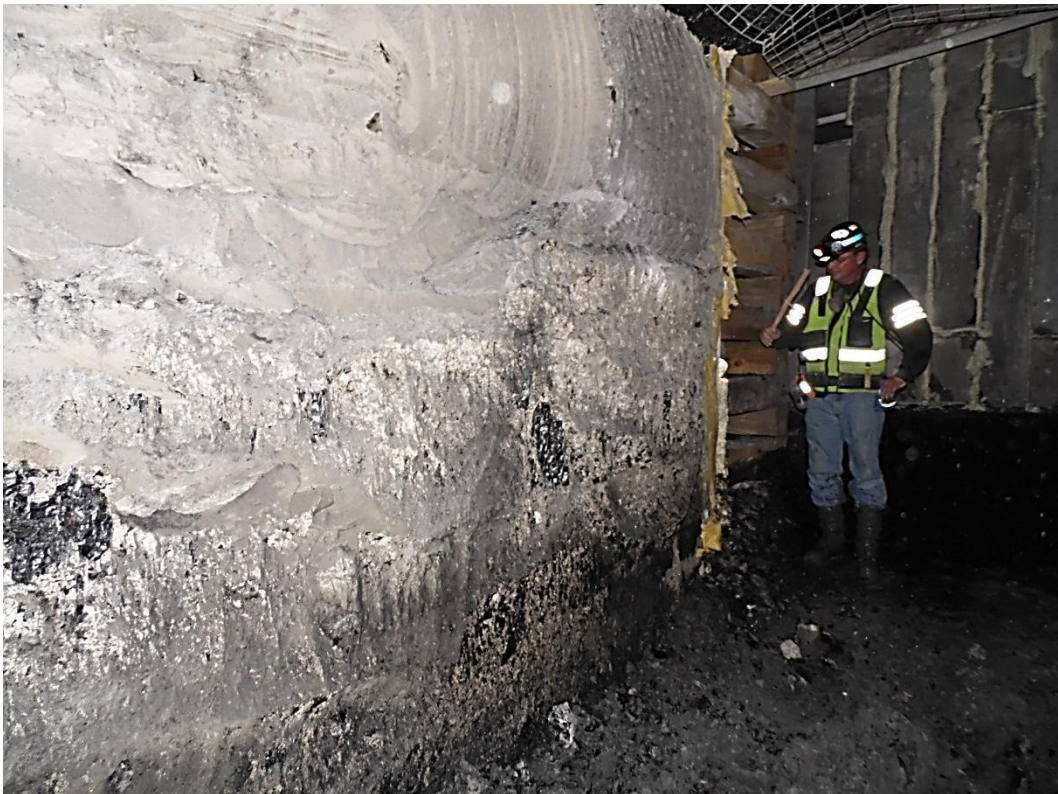
Looking at Phase 1 backfill from Phase 2 development
