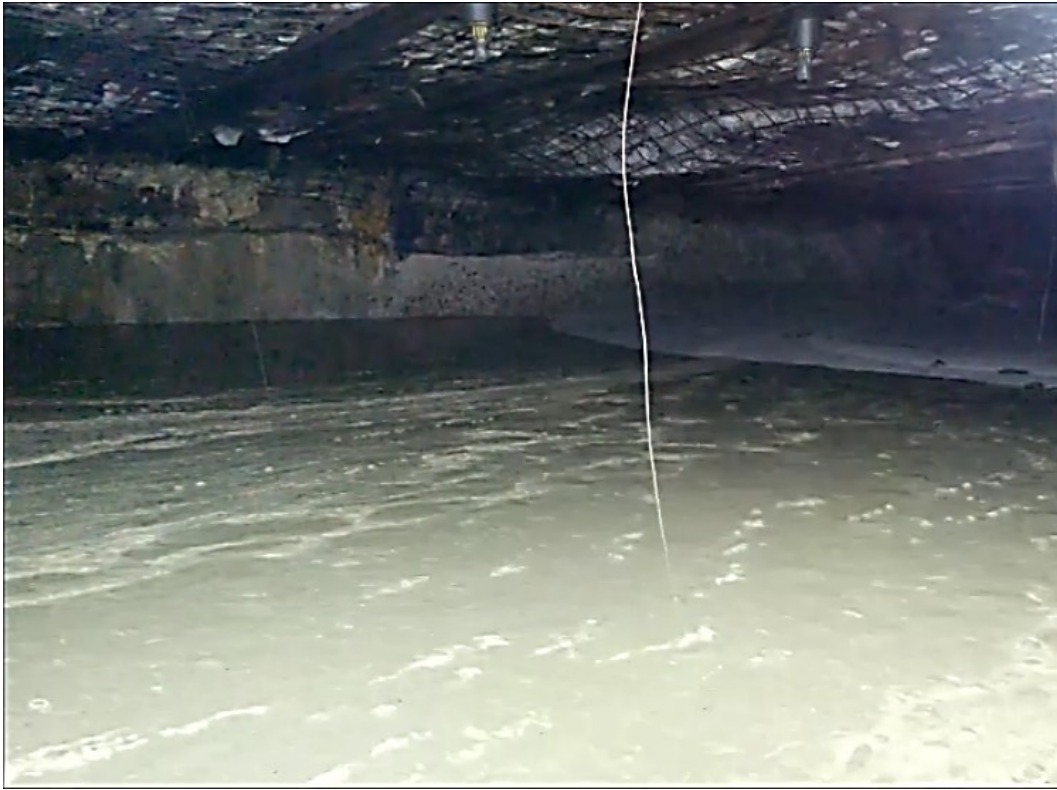
Backfilling 3 Right recovery room
