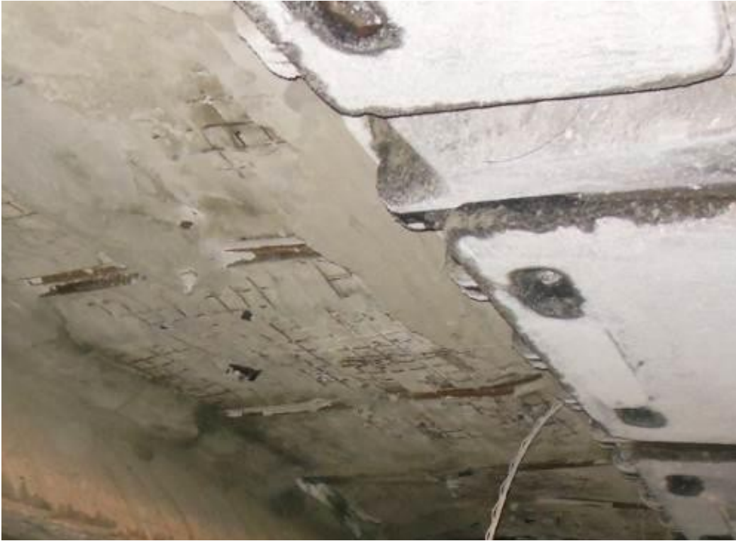
Exposed bolts, channel, and steel mesh
