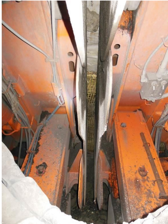
Huesker mesh (yellow) laid down behind the shields
