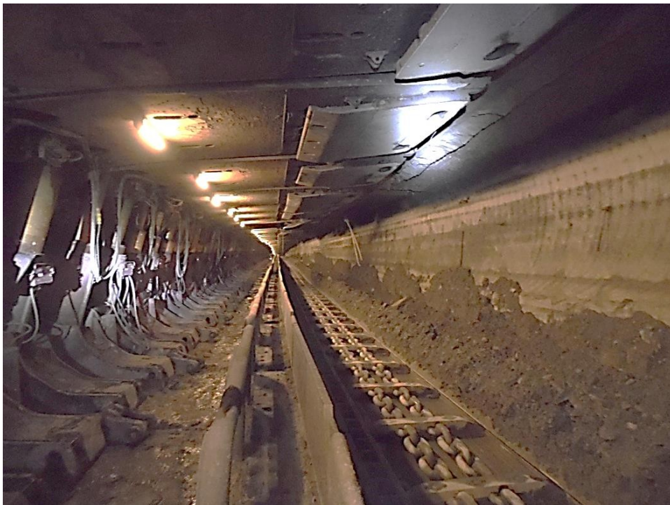
Mining the concrete backfill, no roof spalling. The face is standing straight.
