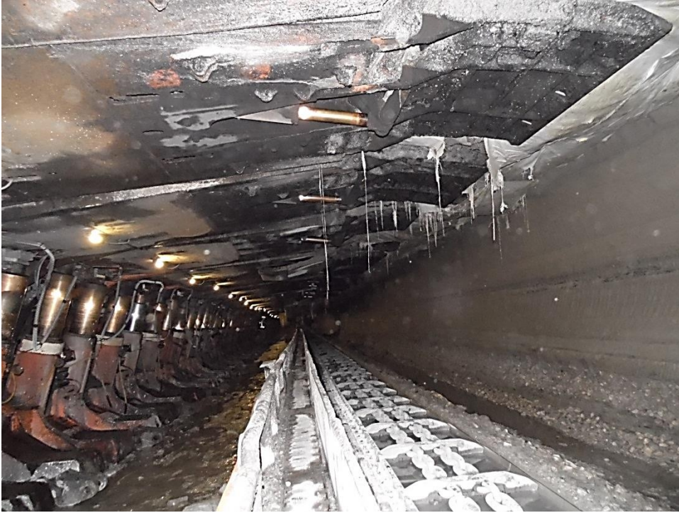
Shield in final position.
