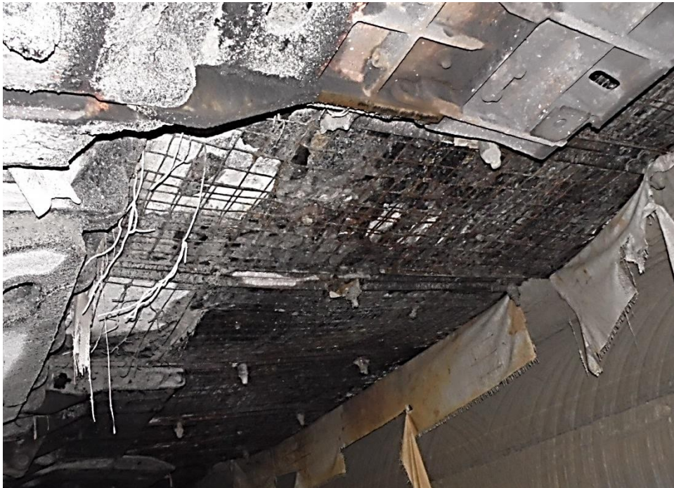
Exposed bolts, channel, and steel mesh.
