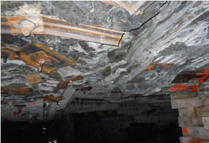
Post-Tensioned Cables
